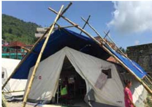
Improvement of tents at Gorkha Hospital © SDC
